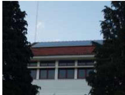
PV systems in the City Hall, schools, and parking coverage (~260kW)
