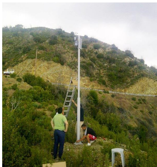
Installation of a meteorological station in the Troodos mountains. Credits: LIFE CALCHAS project
